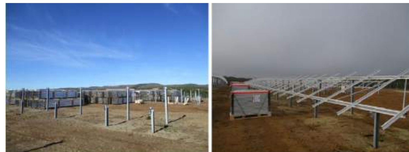
Figure 264 : Assemblage des structures – Q ENERGY France
